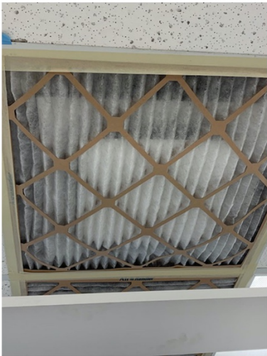
Figure 3. Air filters taken from Dr. Salazar's lab in rooms 442C and 442D. Pictures were taken on September 6, 2021 before the cleaning of the air ventilation system started in September 7, 2021. Pictures of the filters in rooms 442D and 442C show the blackened filter paper and black particles of diverse sizes.
