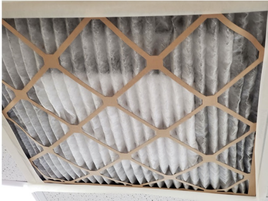
Filter covering the vent in the ceiling of lab
