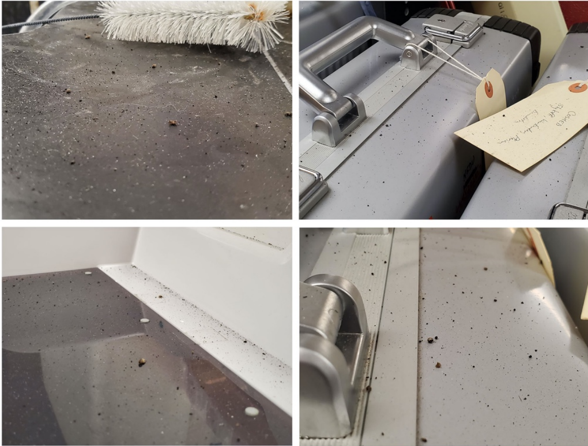
Figure 4. Example of black particles found on surfaces in the Sandels Building. Pictures were taken on September 7, 2021 the day when the cleaning of the air ventilation system started. Pictures show the black particles found on top of benches and equipment in Dr. Kim's lab in Room 440.
