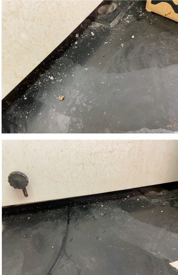
Figure 12. Chemical hood in Room 442G. Example of debris found in the chemical hood located in Room 442G, previously occupied by Dr. Sathe and currently assigned to Dr. Cui. Debris is constantly found inside the hood.
