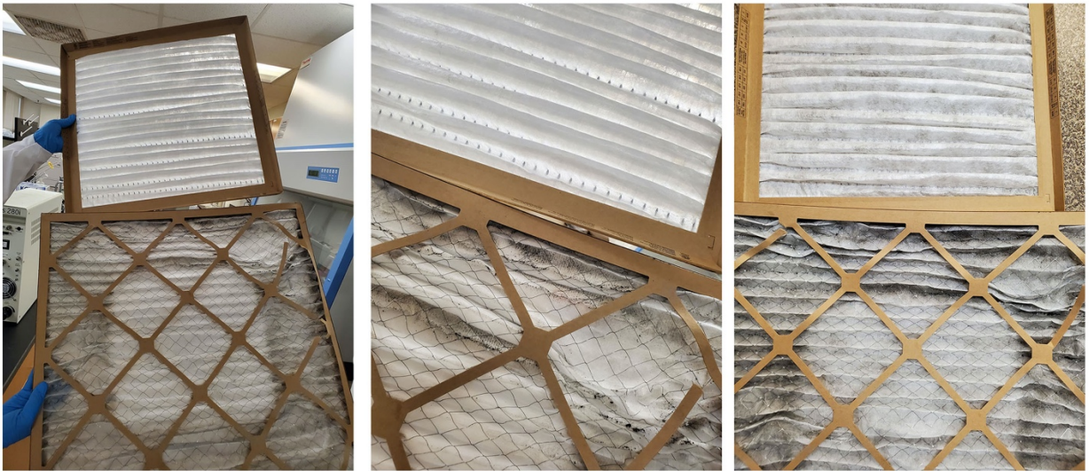
Figure 5. Air filters taken from in Dr. Kim's lab in Room 440. Black particles and blackened paper found on filter covering air vents in Dr. Kim's lab. A) Pictures taken before the filter was removed. B) Pictures comparing the appearance of the filter taken from the lab (bottom) and a new filter (top). The pictures were taken September 7, 2021.
