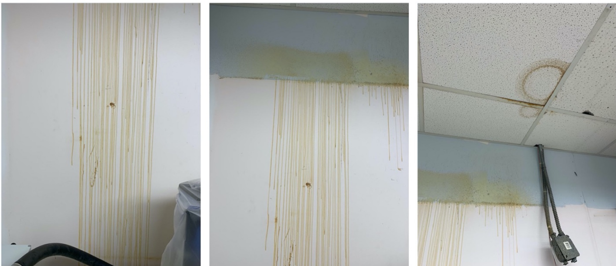
Figure 11. Room 442E Sandels building. Pictures show the condition of the wall where the chemical hood in room 442E was placed. Marks of a yellow liquid are a testimony of what was present inside of the hood.
